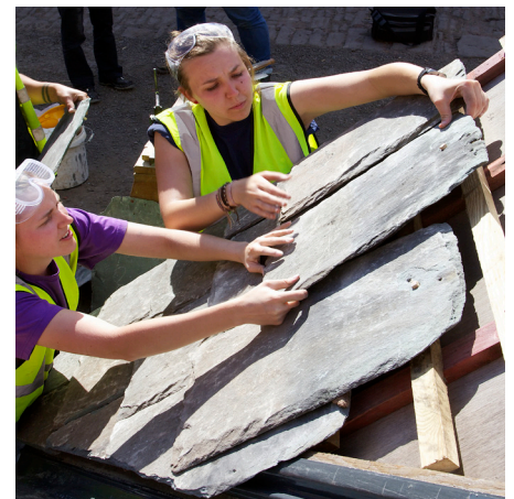
STUDENTS CREATING A SLATE ROOF
